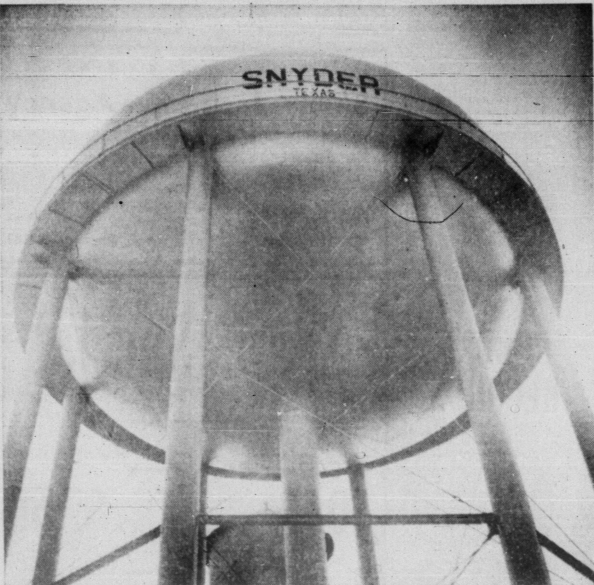
TIMELY ADDITION —This half-million-gallon elevated water storage tank became a timely addition to Snyder's water distribution system today as a heat wave kept the area sweltering. The City Council approved final payment on the contract for the tank last night and the new reservoir was slated to go into service today. (Photo by Jackson)
