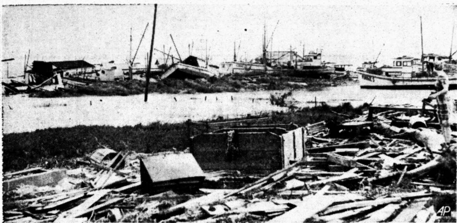
A week end gulf storm which swept 200 miles of the Texas coastal country left these wrecked shrimp boats and debris littering the shores of Palacios, Texas. Some of the small craft were sunk, others left tilted on sandbars.
