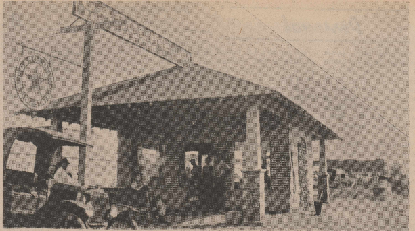
FIRST FILLING STATION
