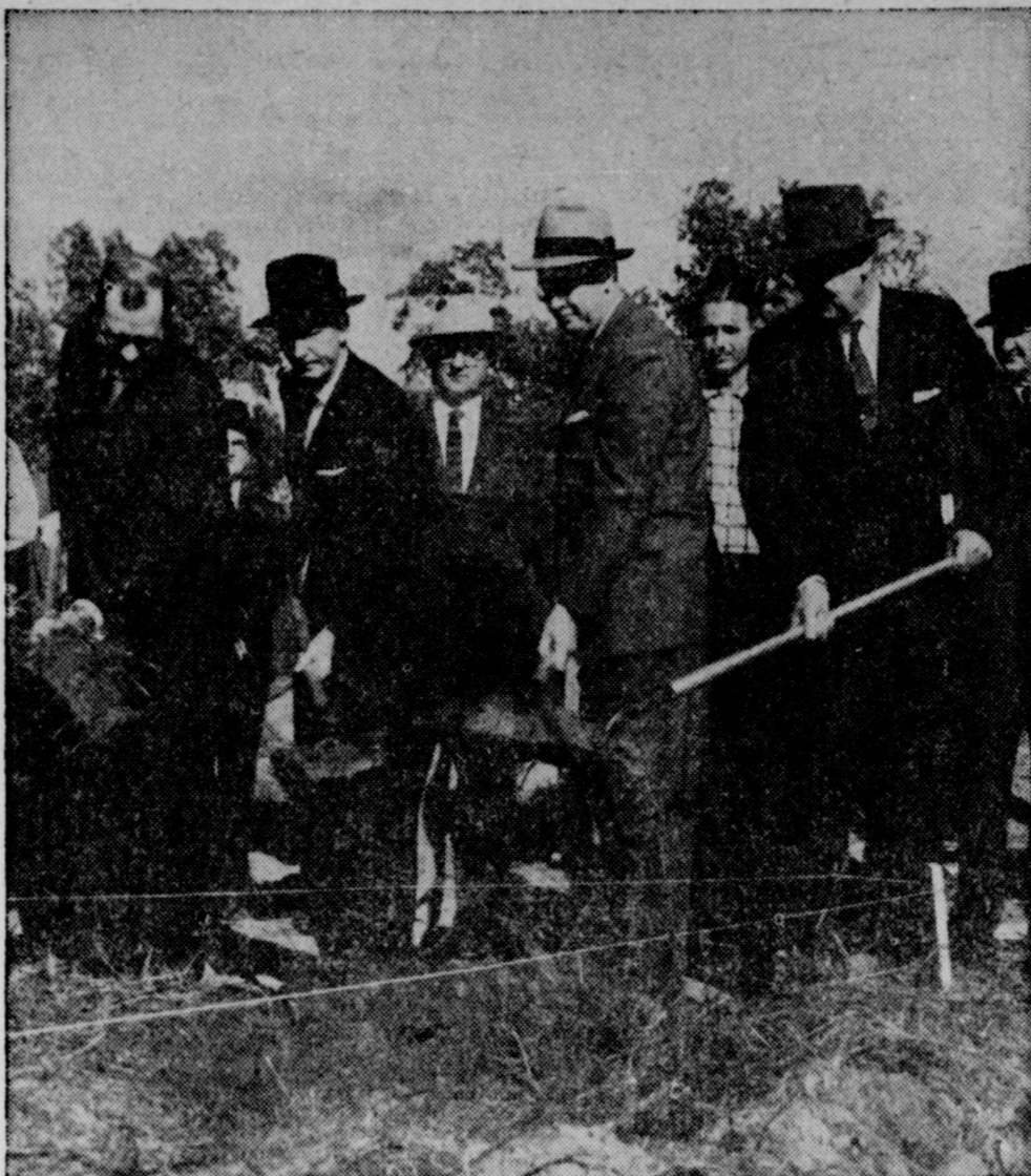
BREAKING GROUND near Vivian, La., for the new 1553-foot TV tower of KCMC-TV Channel 6, Texarkana, are four mavers. Left to right: R. P. McElroy, Texarkana, Texas; Clyde Fant, Shreveport; Haskell Hay, Texarkana, Arkansas, and Jake Cameron, Bossier City. The new tower, expected to be ready in early 1961, will serve 1 1/4 million people in the Ark-La-Tex. The tallest tower in the South, it will be the fifth tallest man-made structure in the world.
