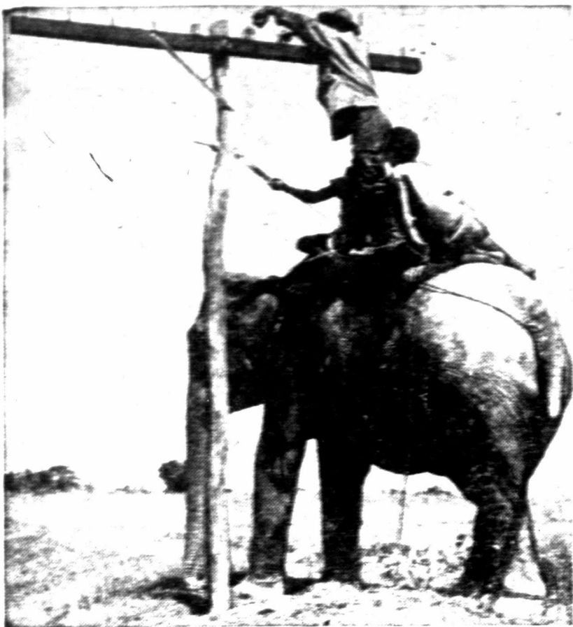
A member of the American signal construction outfit is shown repairing a line from the back of an elephant. These slow-moving patient animals are used to very good advantage in the swamplands at Assam, India, by native and Allied troops. The signal corps, under unusual conditions, have managed to install and keep open communication lines.
