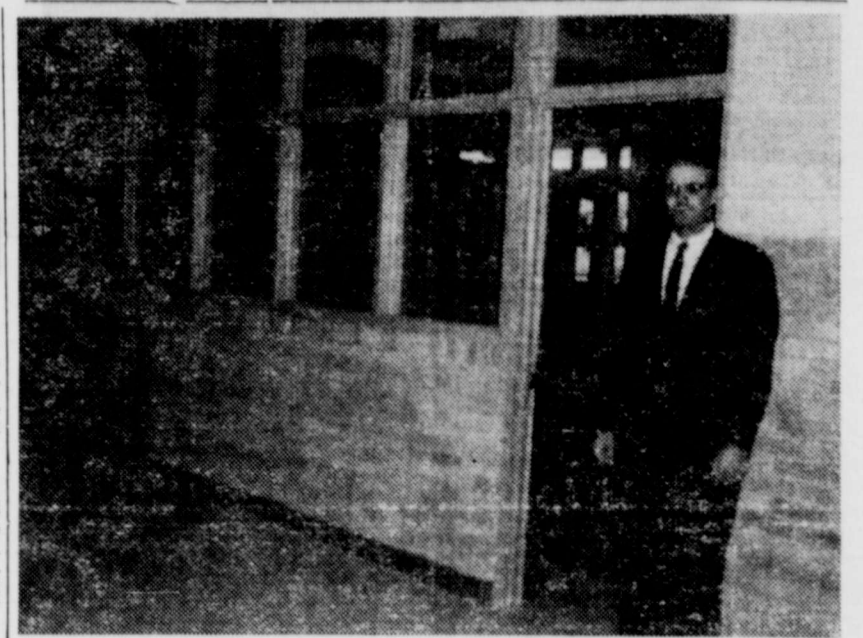
JUNIOR HIGH PRINCIPAL —Gid Adkisson, Principal of Abernathy Junior High, is pictured here standing at the door of his office in the new Junior High building. The new building features brick walls, terrazzo corridors, vinyl asbestos tile floor in classrooms, and semi-open stack library which is air conditioned.—(Staff Photo).
