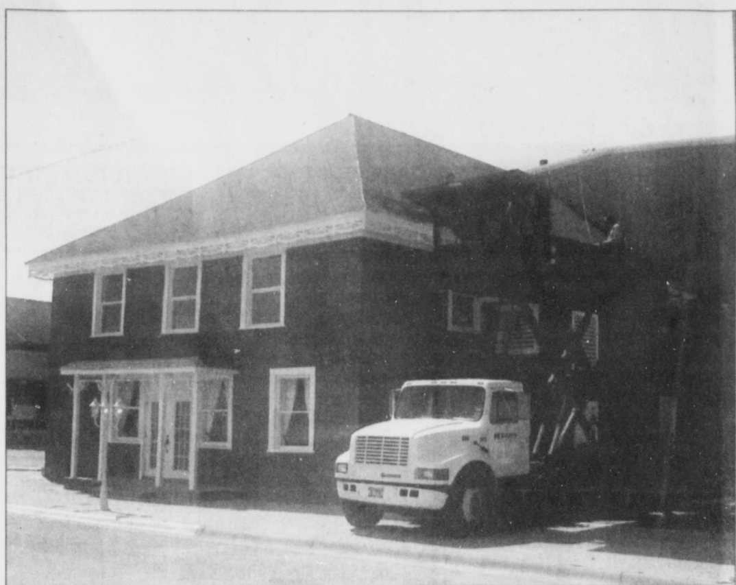
THE OPERA HOUSE sports a new roof as workers put the finishing touches on repairs to the building which was weather damaged in 2009. Photo courtesy of City Hall
