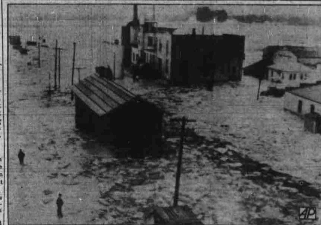
Sixty per cent of Sebawaing, Mich., was covered with water and drifting ice cakes as the Sebawaing river, its mouth clogged by ice, left its banks. This picture shows the flooded Pere Marquette railroad yards at Sebawaing. Flood waters gave trouble in other parts of Michigan, Wisconsin and Ontario.
