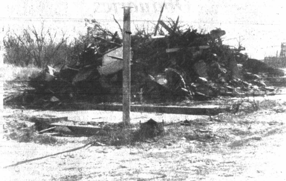
BUILDING RAZED —Another community "eye sore" is soon to disappear as city crews demolished the old station building at Waco Street and East Highway 80, this week.
