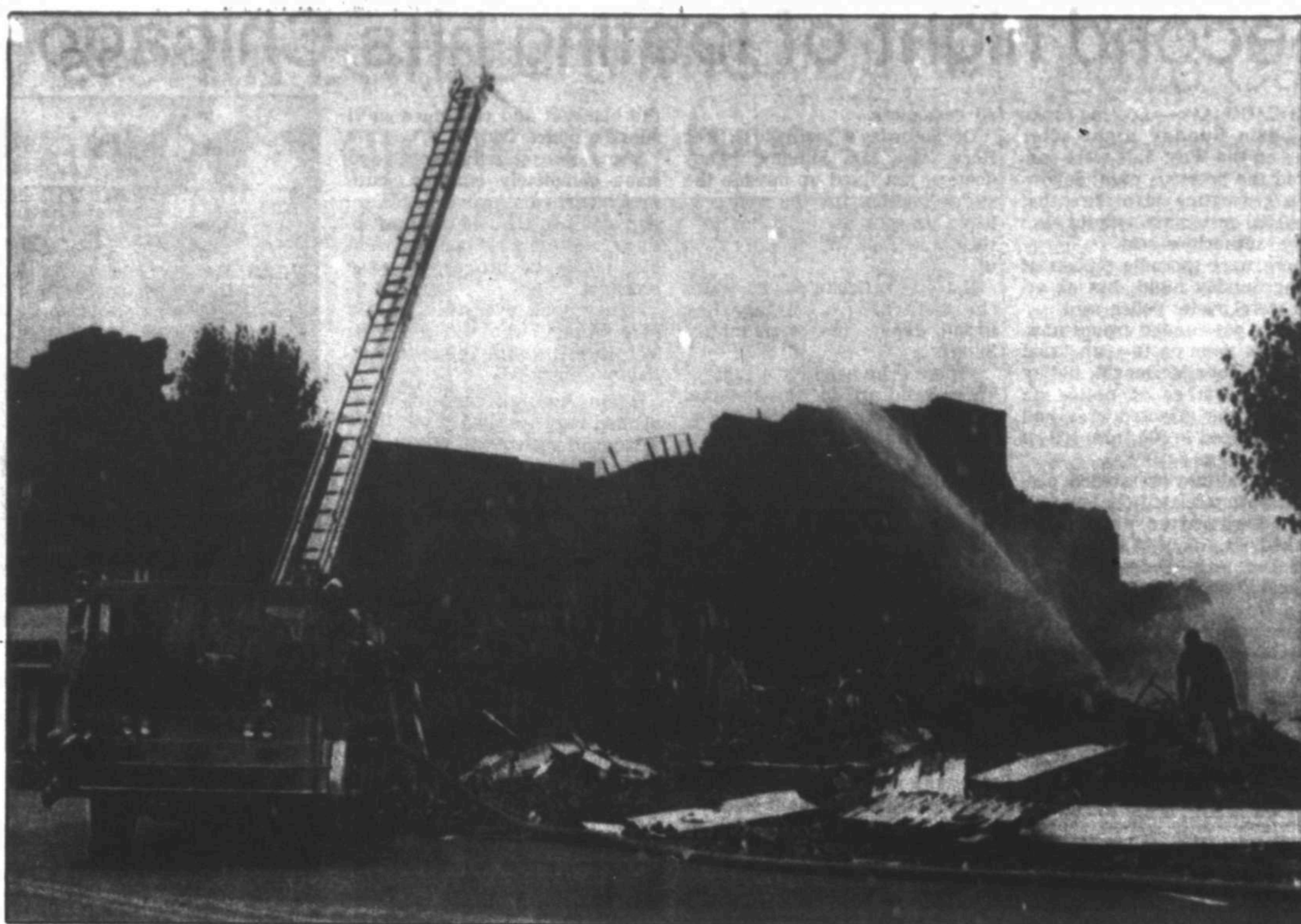
Firemen spray buildings in downtown Monroe, N.C., Sunday after an explosion and fire damaged several buildings.
