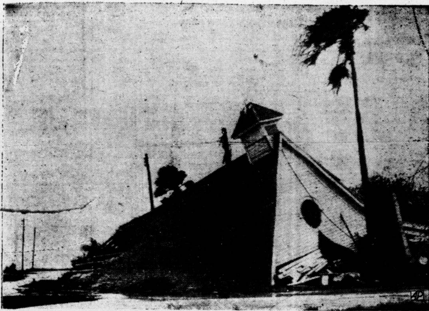
STORM FLATTENS CHURCH — A tropical hurricane which ravaged the Gulf Coast of Texas demolished this church at Port Lavaca. Property and crop damage was estimated at millions of dollars. (AP Wirephoto).
