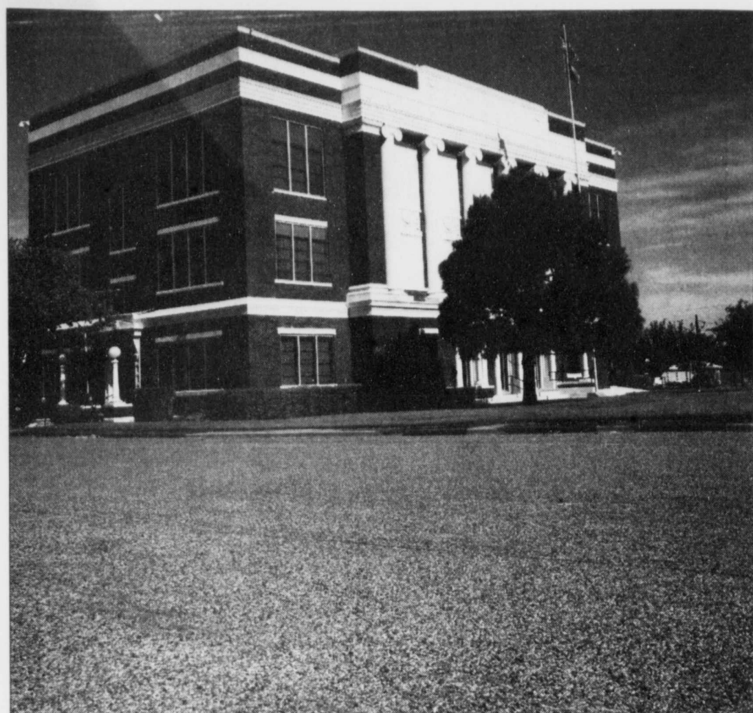
CLOSED FOR REPAIRS — an empty parking lot at the county courthouse reminds residents that the courthouse will be closed until further notice for repairs due to water damage and asbestos abatement.
