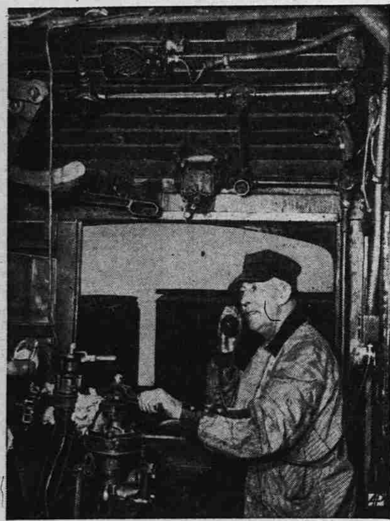
TRAIN RADIO—Sitting in the locomotive of a New Haven Railroad freight train, Engineer John J. Desmond talks with the freight conductor on the caboose a mile to the rear in train radio experiment. Loud speaker is on cab ceiling.
