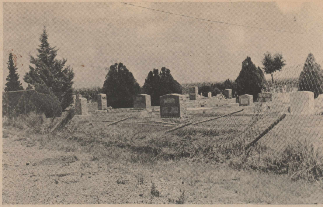
DAMAGED FENCE AT OLTON CEMETERY
