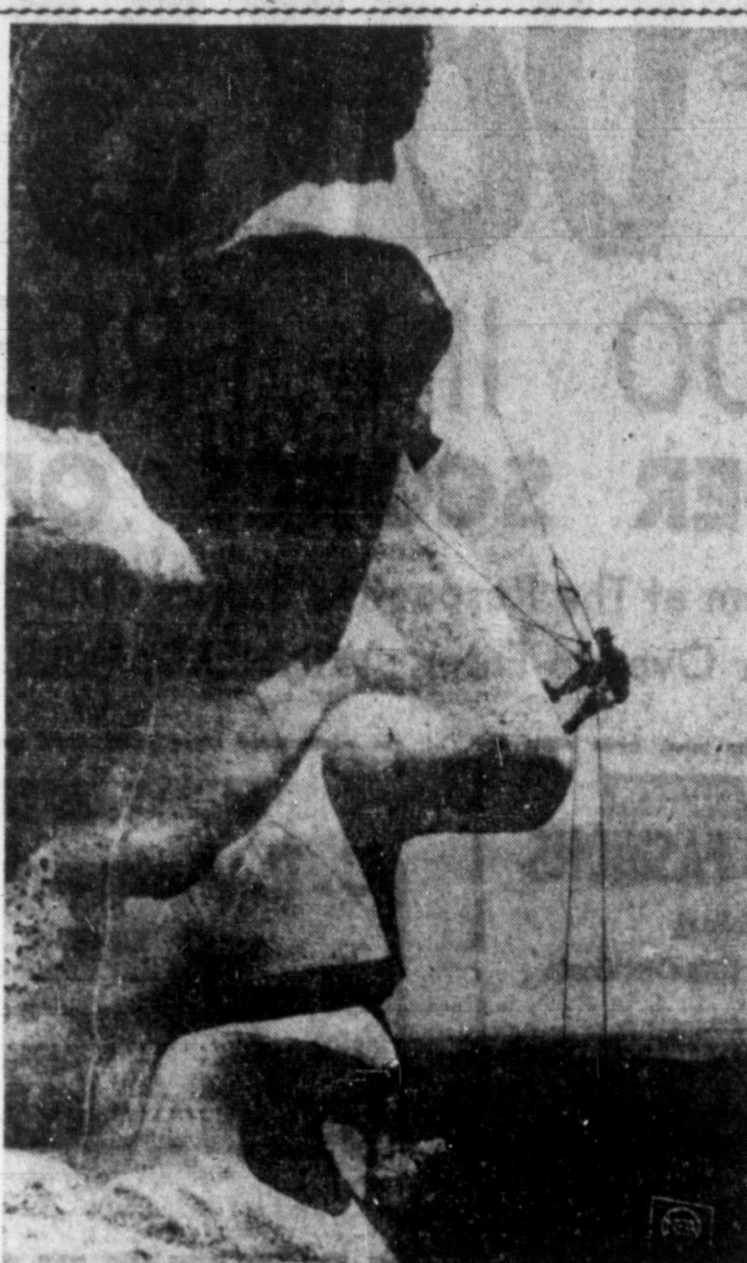
FACE LIFT—Mike O'Mera traverses granite face of Abraham Lincoln while repairing cracks at Mt. Rushmore, S.D.
