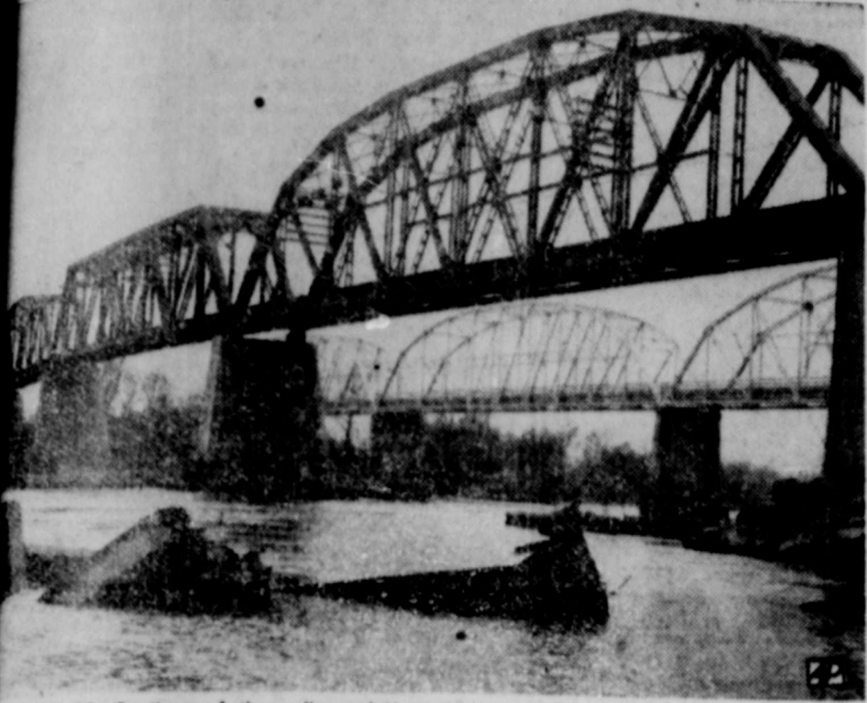
OR DEFENSE—Portions of the collapsed Katy Railroad bridge near Denison are to be salvaged for the national defense drive. Visible in the foreground are the old bridge that washed out in a flood in 1908. Some old coal cars had been moved onto the bridge to hold it. The cars, too, will be salvaged. (P. Photo)
