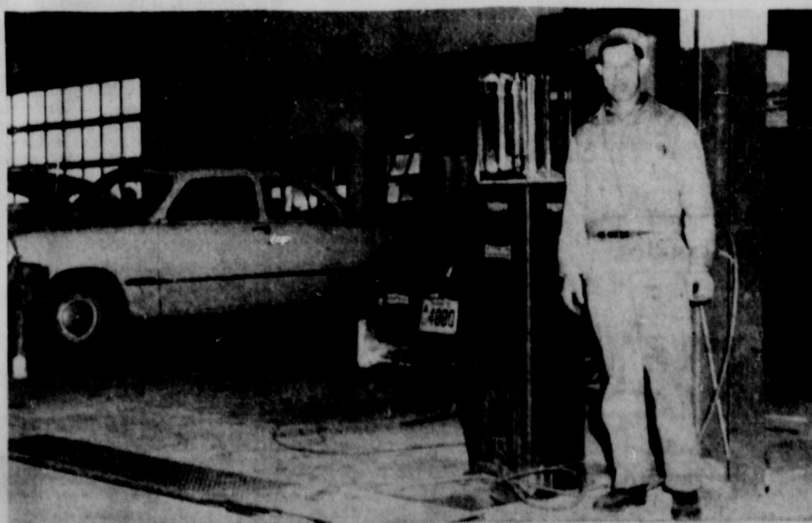
BRAKE TESTER —Nope, it's not a gasoline pump that John Schollenbarger of the A&B Motor Co. is standing by. This is the new Weaver brake testing machine installed last week. It also checks front end alignment. An automobile is driven on the metal platform, the brakes are thrown on, and the tester shoots up four columns of red liquid in glass tubes, showing what each brake registers. This is one of the tests to be applied under the new Texas inspection law.
