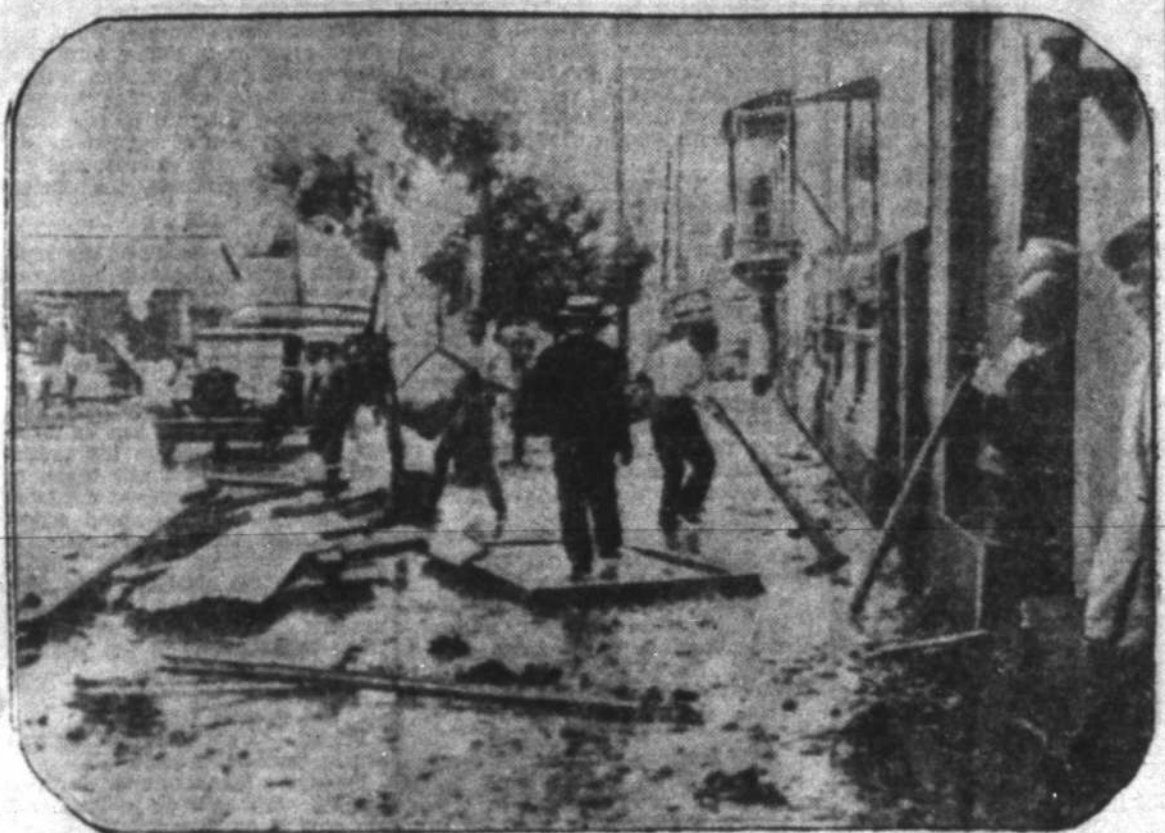
Rushed to the United States by airplane and then distributed by telephoto, the above picture shows a view of a hurricane-torn street in San Juan, Porto Rico. Note the window casings, blown onto the walk.
