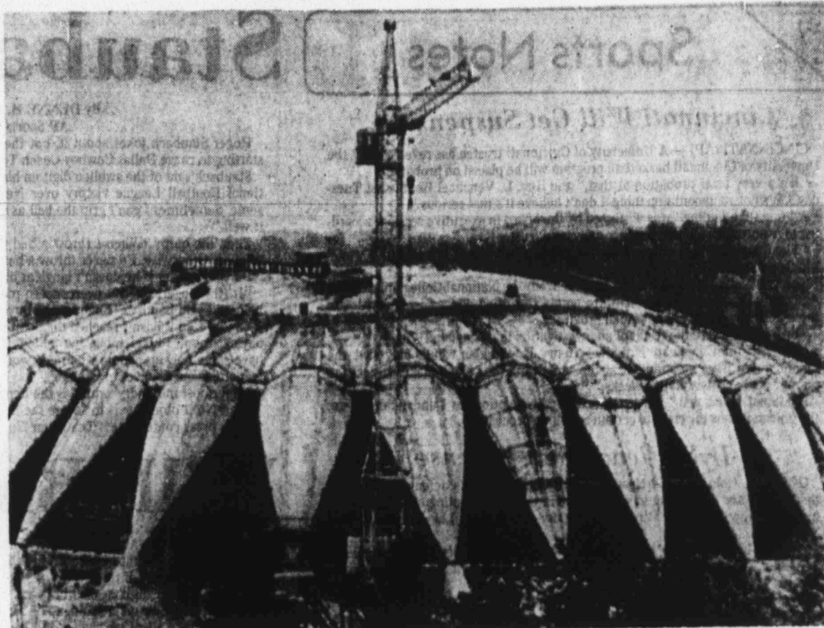
PREPARING FOR THE OLYMPICS — Installation of a "rigidity frame" weighing 500 tons continued in Moscow as workers prepare the Luzhniki sports complex for the 1980 Olympics. The complex will accommodate more than 30 percent of the Olympic program. (AP Laserphoto)
