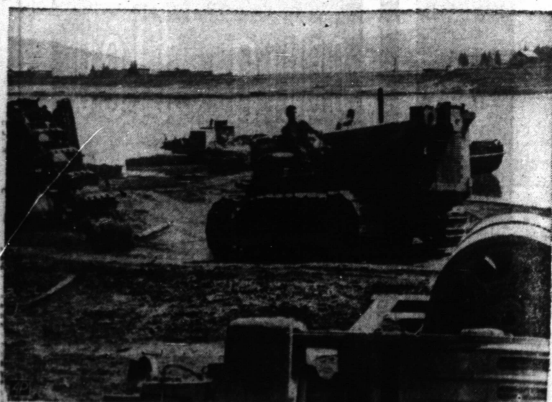
RED OIL OPERATION —Workers move machines along banks of the Lena river for use in the Markov oil deposit area. Two borings have been made in the recently-opened field in Irkutsk province in south Siberian section of the Soviet Union.
