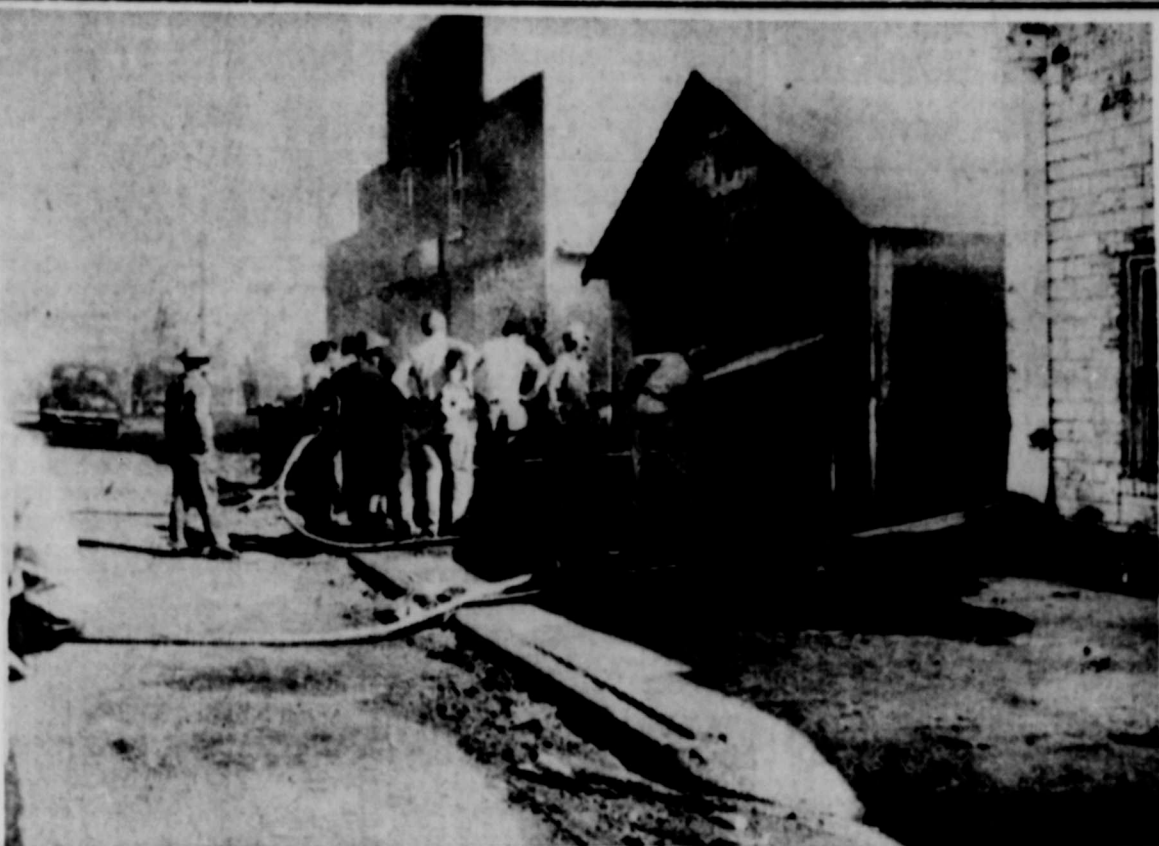
PAINT SHOP FIRE —The interior of this building was badly damaged Thursday in a fire which started when an automobile backfired. A. W. Belt, owner of the shop, was pouring gasoline into the carburetor of the car and as O. C. Rickard stepped on the starter, flames shot out and set the gasoline on fire. The automobile was badly damaged, and the fire spread rapidly throughout the interior of the building. No one was injured.
