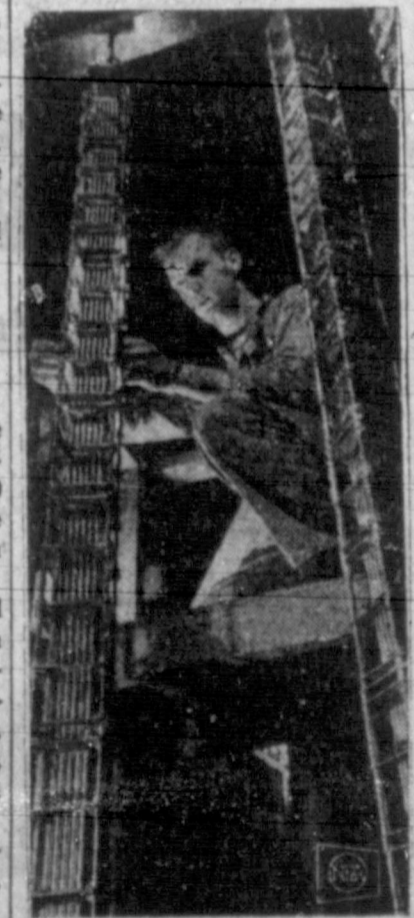
ATOMIC PILER—Technician Lester Race checks fuel bundles in Yankee Atomic Electric Co.'s nuclear plant at Rowe, Mass. A second fuel charge of 25 tons of uranium oxide will be installed in the reactor early this spring.
