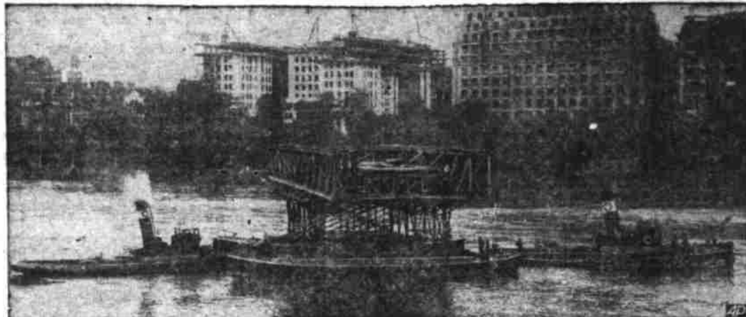
MAN WAITED FOR TIME AND TIDE in setting two 110-ton navigation spans in position near site of the new permanent Waterloo bridge at London. With hawsers steadying them, the spans—one of which is shown resting on barges—sank inch by inch as the tide ebbed until ends of the horizontal girders rested accurately on the greased tops of river piles below.
