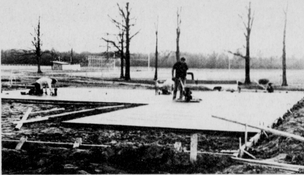
NEW BUILDING —Now under construction is a new building for the Rivercrest FFA Chapter to replace the one that burned. The chapter is now housed in the Vocational Agriculture Building at Talco Junior High School, and students are bused back and forth for classes. (Staff Photo)
