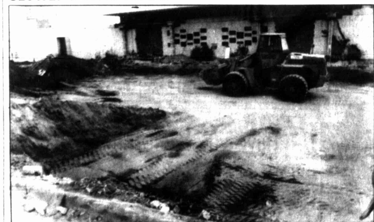
Herald photo by Tim Appel A bulldozer removes dirt from a pit behind the old Bluebonnet Savings building Tuesday as work is underway in renovating it to become the new Howard County Library. The building will be expanded into the area, formerly a parking lot.
