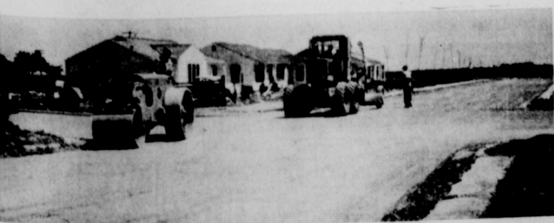
Bill Wilson Crew On Paving Job
