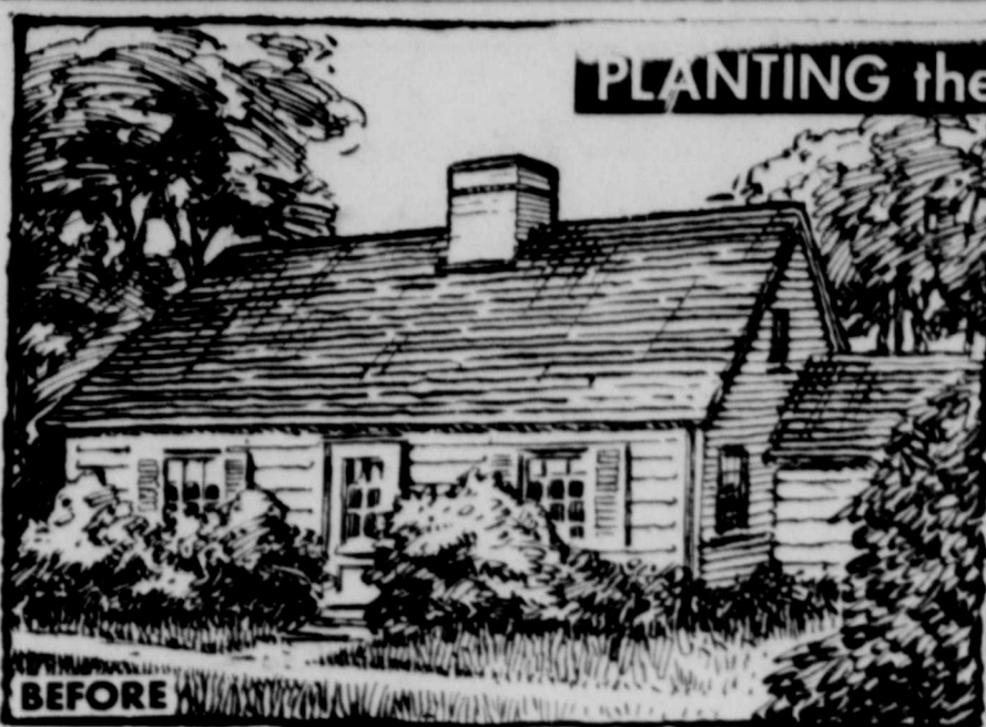
PLANTING that wasted $100. It looked pretty for a couple of years when there were leaves on the bushes, but during the winter it added no color to the house. As time went on it was necessary to trim constantly to keep the bushes from obstructing the windows and spreading over in front of the house.
