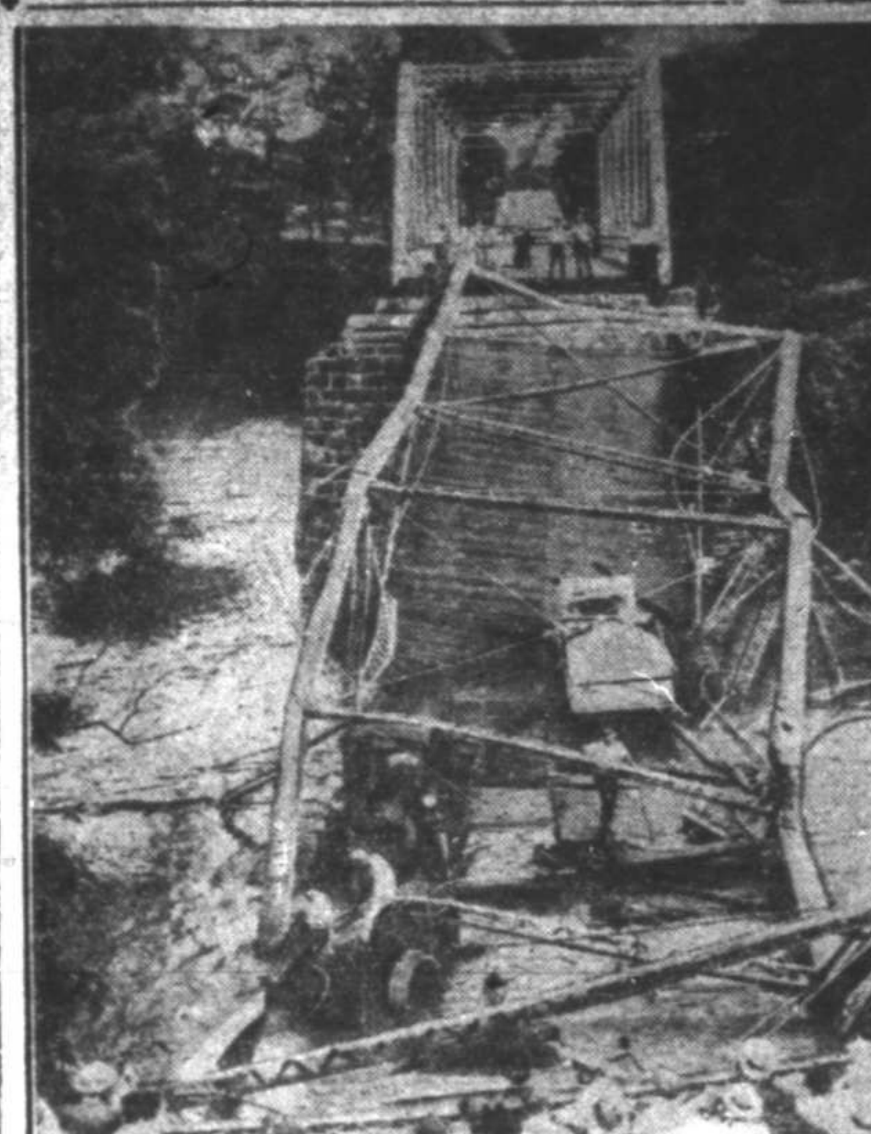
Three men were killed and six hurt when this steel bridge over the Monocacy river on the Washington highway near Frederick Md., collapsed and hurled workmen and trucks 20 feet into the swollen water. The men were repairing the structure when a heavy truck drove onto the bridge causing the collapse.
