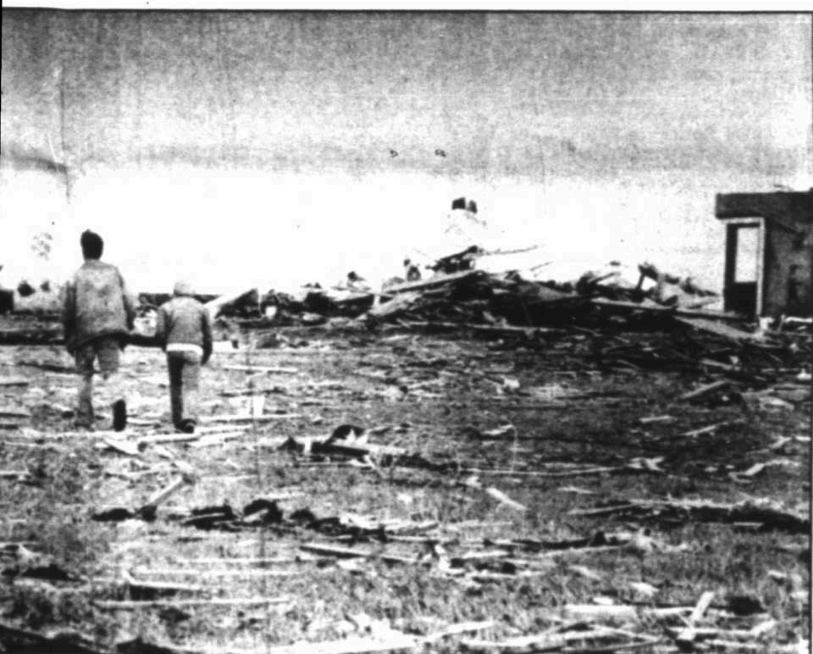
Two Sweetwater residents, left, walk through the debris after the tornado touched down Saturday morning, leaving a path of destruction a half-mile wide and two miles long.
