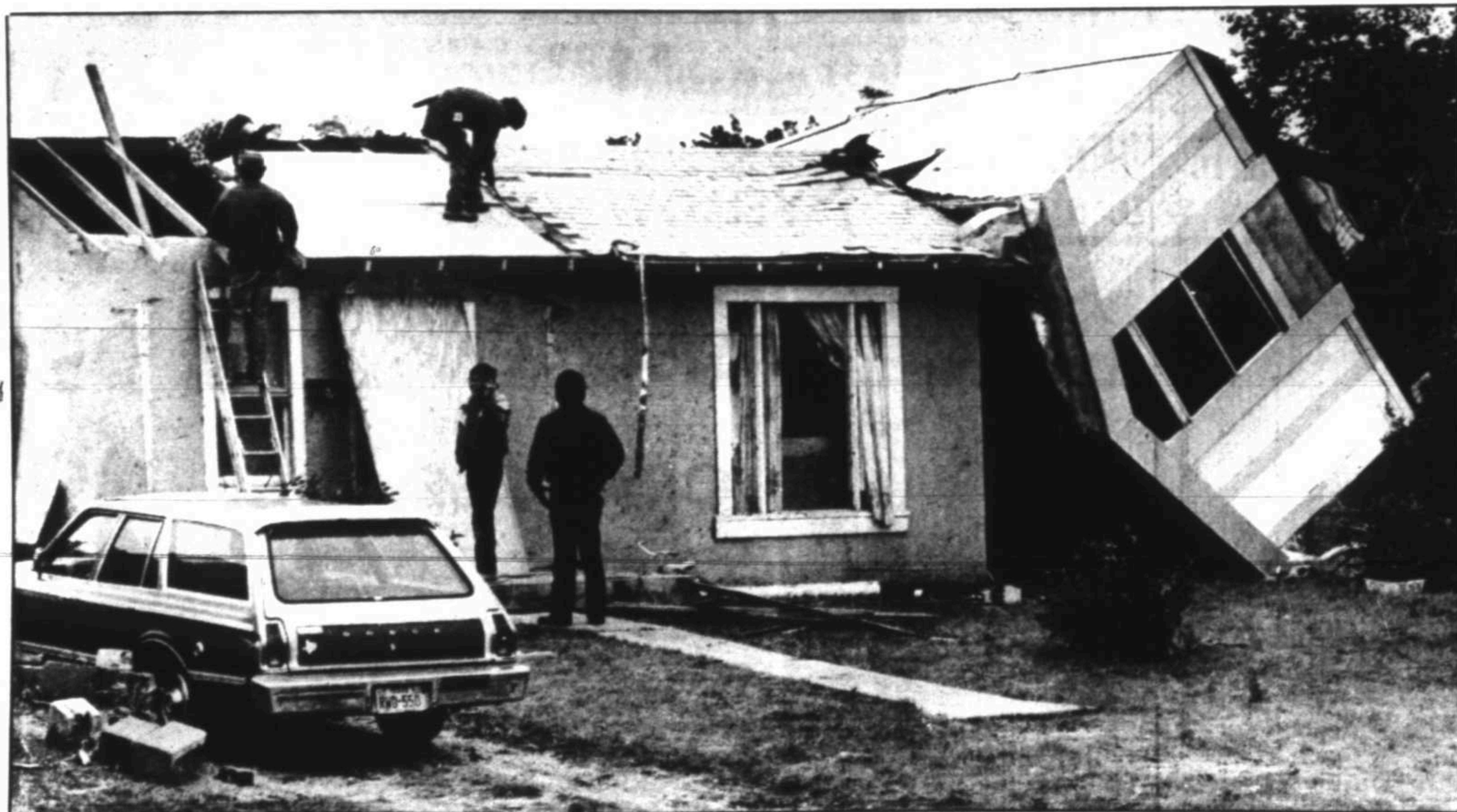
Within hours after the tornado struck, many Sweetwater residents were busy digging out and repairing the damage.
