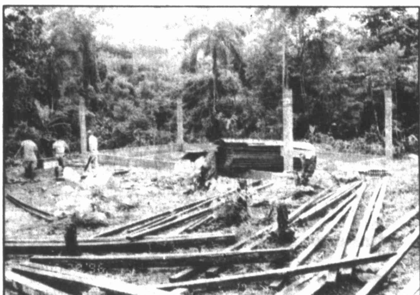
This is the beginning stage of the building with the concrete poured and the wood ready to be put up.
