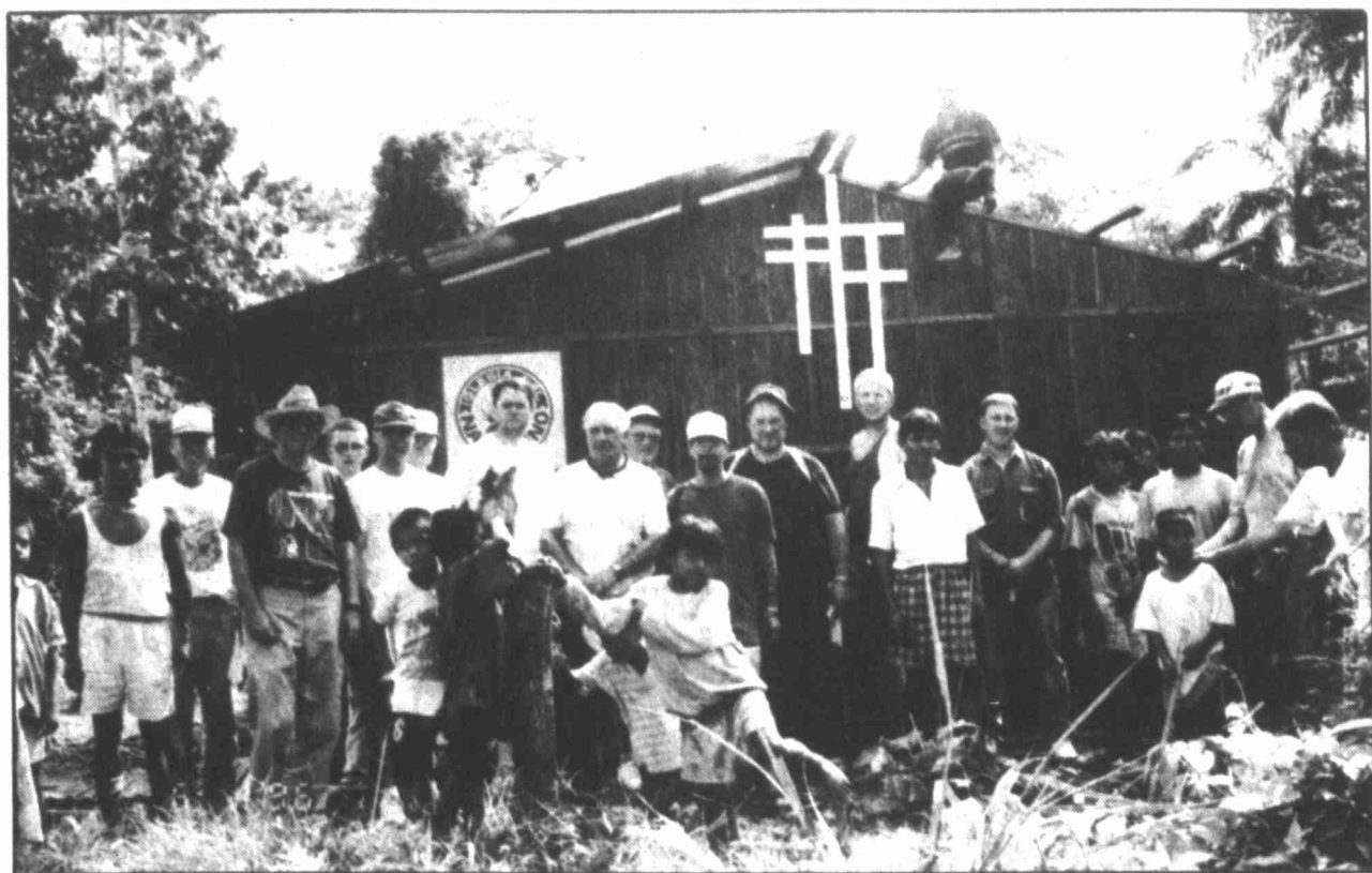
The First Church of the Nazarene group stand among the Aguarunas in the Amazon jungle. The Big Spring entourage traveled to South America to build a church for the villagers.
