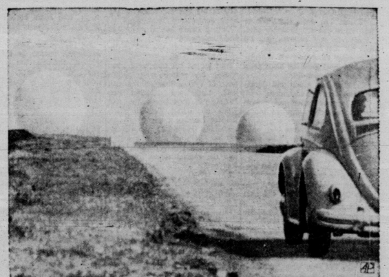
BALLS IN THE MOOR —Motorists driving through Fylingdale Moor, Yorkshire, England, come upon a strange sight—huge spheres on the horizon. They're 154-foot tall radomes, enclosing tracking radar transmitters of the missile early warning station.
