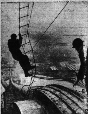
HIGH WORK —Steelworker climbs down from tower to catwalk after disconnecting cable-spinning equipment on new bridge spanning Firth of Forth in Scotland.
