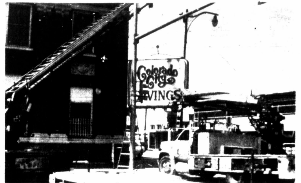
A FACELIFT was given to the Colorado City Savings and Loan building Wednesday afternoon by the installation of a new sign. The large red, white and yellow sign is a bright addition to the downtown area.
