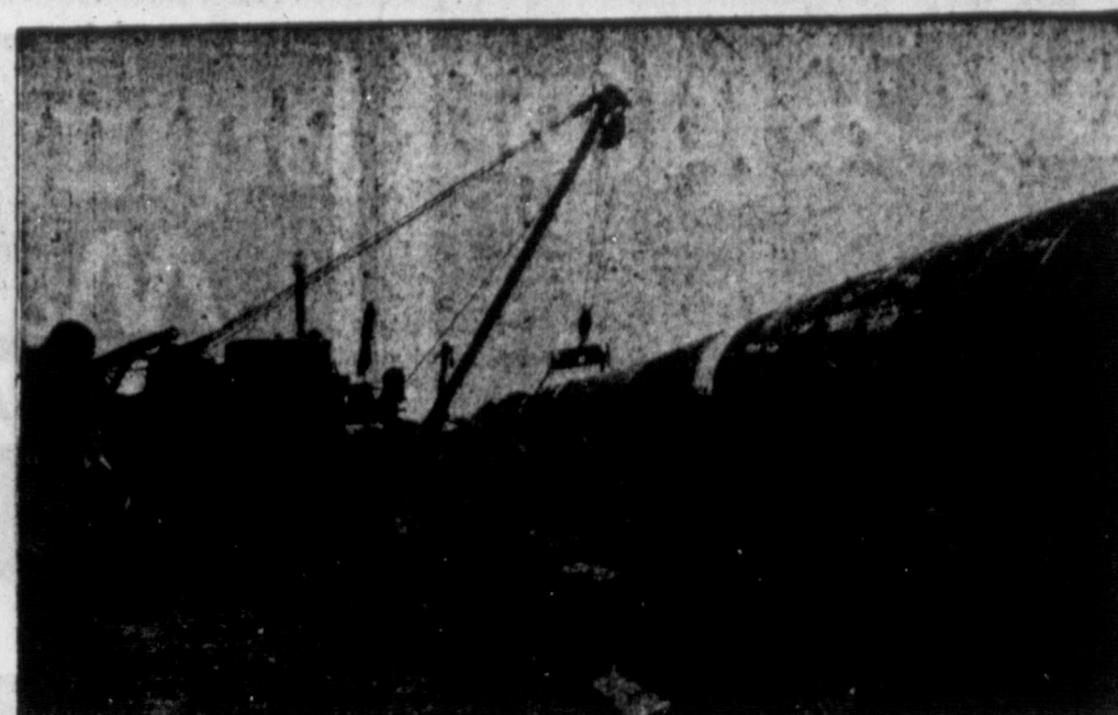
Wrapped with corrosion-resistant material, a section of new 26-inch gas pipeline is readied for lowering into a ditch near Tonganoxie, Kans., as part of Cities Service Gas Company's $14 million construction program for 1964. The new pipe, made of quarter-inch steel and weighing nearly 70 pounds per foot, replaces a smaller pipeline and increases the capacity of the gas company's system serving northeast Kansas.
