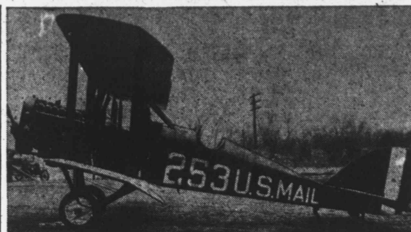
THEN—This DeHaviland was built for the First World war, became a mail plane when the post office department started the first coast-to-coast airway in 1920. Equipped with a 400-horsepower Liberty motor, it carried its pilot and up to 400 pounds of mail at a cruising speed of around 100 miles an hour. It was an open cockpit job—as was the ancient Model T in the background!
