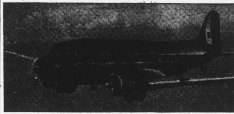
NOW—This United Air Lines Mailliner, with its two 1,200-horsepower Pratt and Whitney Wasp engines carries two pilots, a stewardess, up to 21 passengers, baggage, and approximately 2,000 pounds of mail and express at a cruising speed of 200 miles an hour. It flies coast-to-coast overnight.
