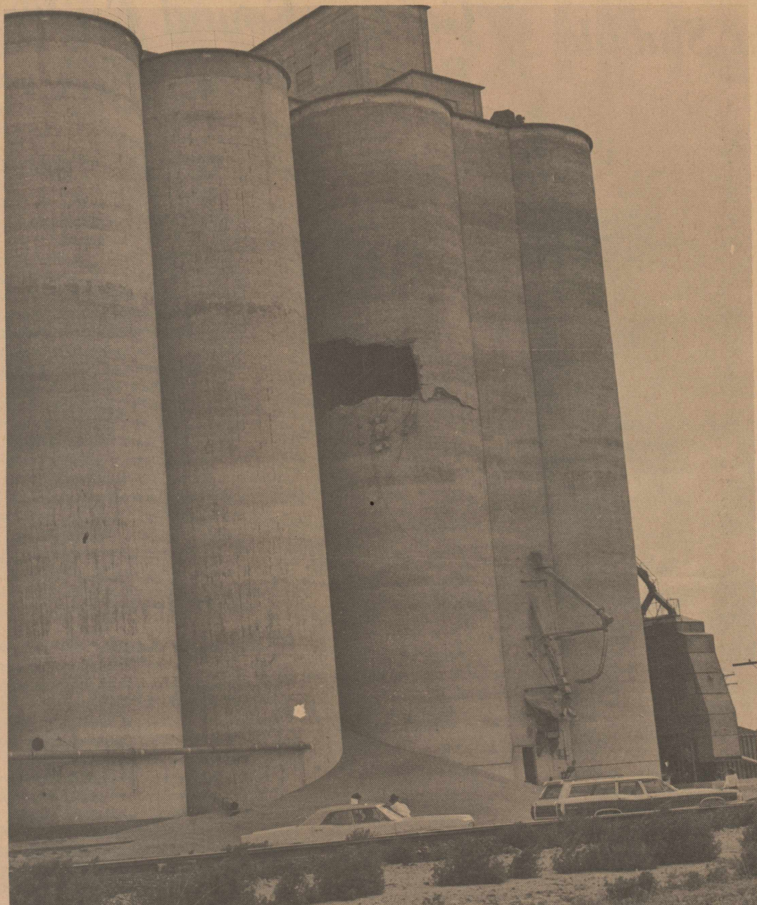
ELEVATOR WALL FAILS---Kerrick Grain Co., located on Highway 287 northwest of Stratford on the Oklahoma line, was struck by misfortune for the second year in a row late Monday afternoon. Part of the walls of one of the tall concrete tanks of the elevator fell away leaving a gaping hole big enough to drive a small truck through and letting an estimated 30,000 bushels of wheat fall to the ground. The tank which collapsed was filled all the way with newly-harvested wheat. Cone Donelson, owner, said there was no explosion. He said about a half-hour before the wall fell that workmen saw a big bulge coming at the place where the concrete fell away. A similar fate befell the elevator last summer on another tank on the same elevator.
