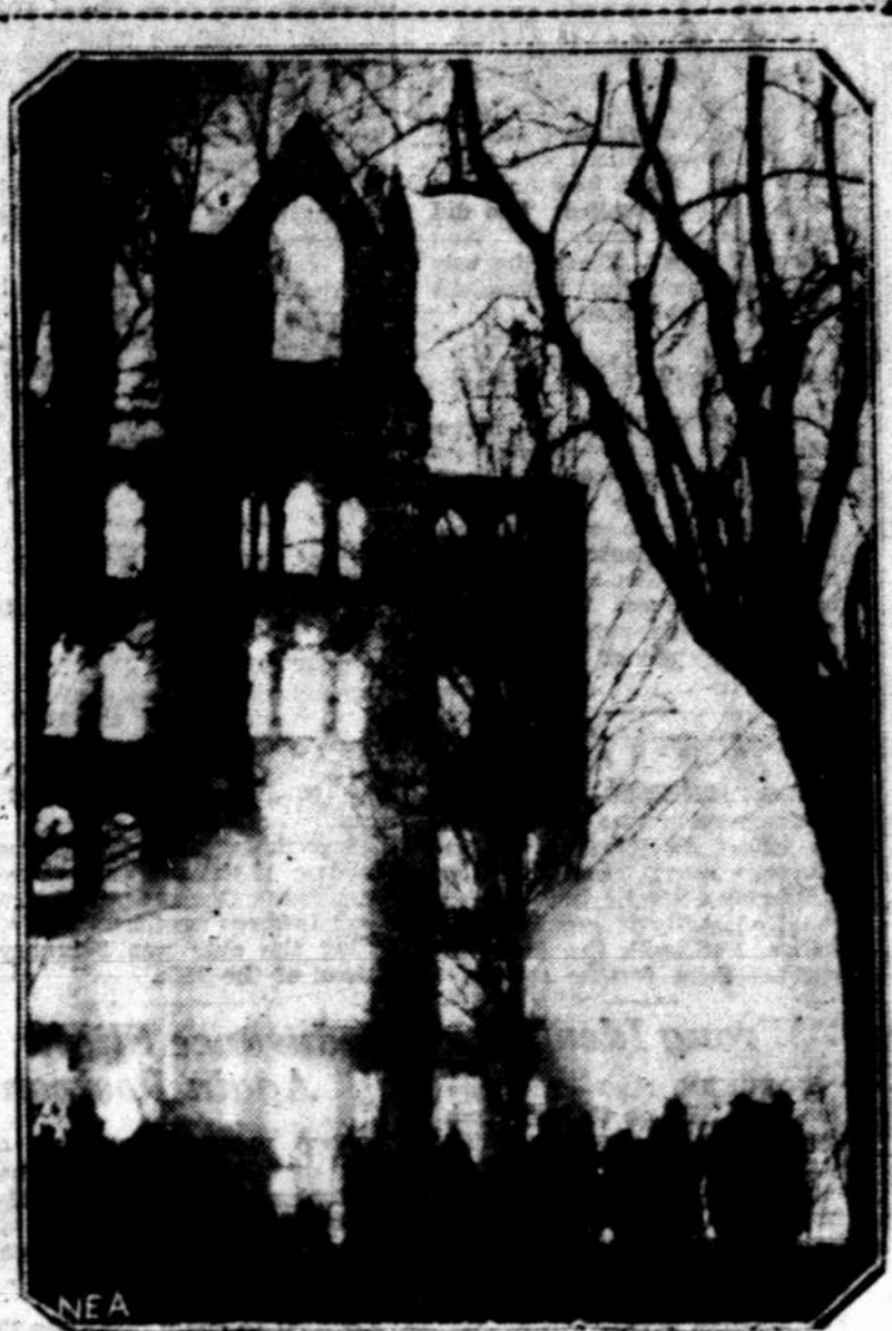
Undergraduate volunteer firemen at Villanova College, Philadelphia, worked overtime while flames they were powerless to stem destroyed the main building, pictured above, and damaged a nearby monastery and church.
