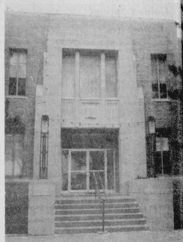
Workers are busy sand-blasting the court house this week!
