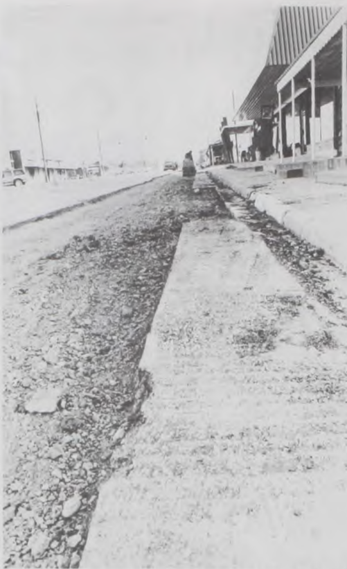
Torn up pavement on the east side of Main Street has crippled sales of many local businesses during the past few weeks. Patching the street where new water lines have been laid should be completed for this weekend's Germanfest. Photo by Janie Hartman
