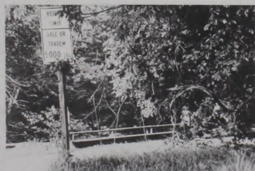
The bridge on west Eddy Street will be closed next Wednesday, April 28 waiting for a replacement. It has been declared unsafe.
