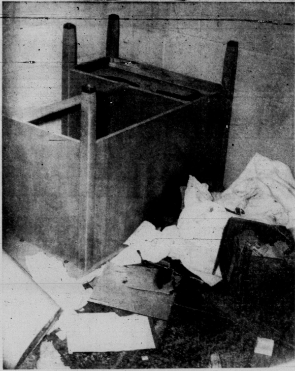
HANDIWORK OF VANDALS —This destruction of property occurred sometime during the weekend at Northeast Elementary School, one of three buildings entered by burglars. The Northeast school sustained most damage, with broken windows, smashed desks and other vandalism. The West Elementary School building and the Boys Club Building also were burglarized over the weekend.
