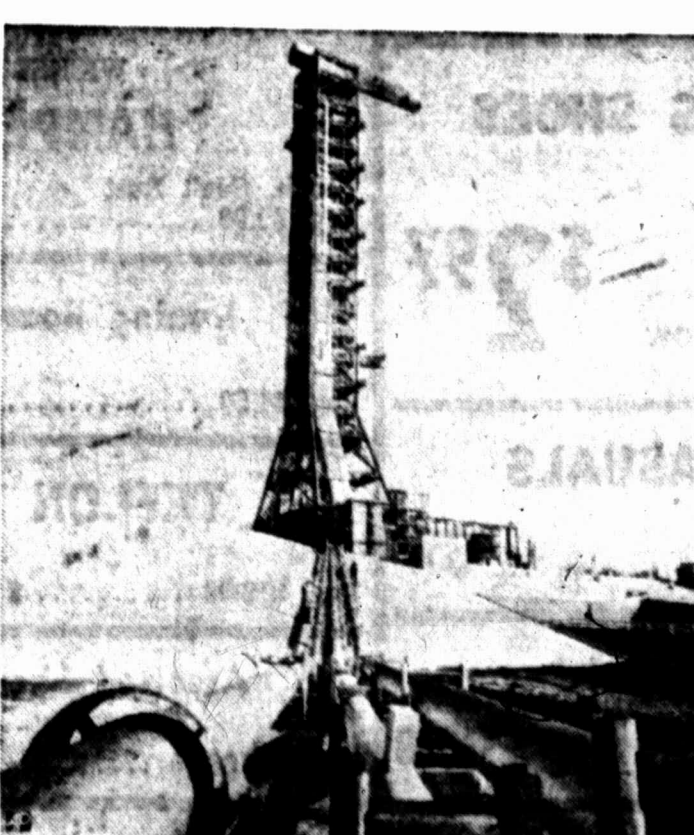
SPACE PLUMBING —Bendix technicians send nitrogen gas through these pipelines to clean fuel lines in Apollo moon rocket tower at Cape Kennedy, Fla.
