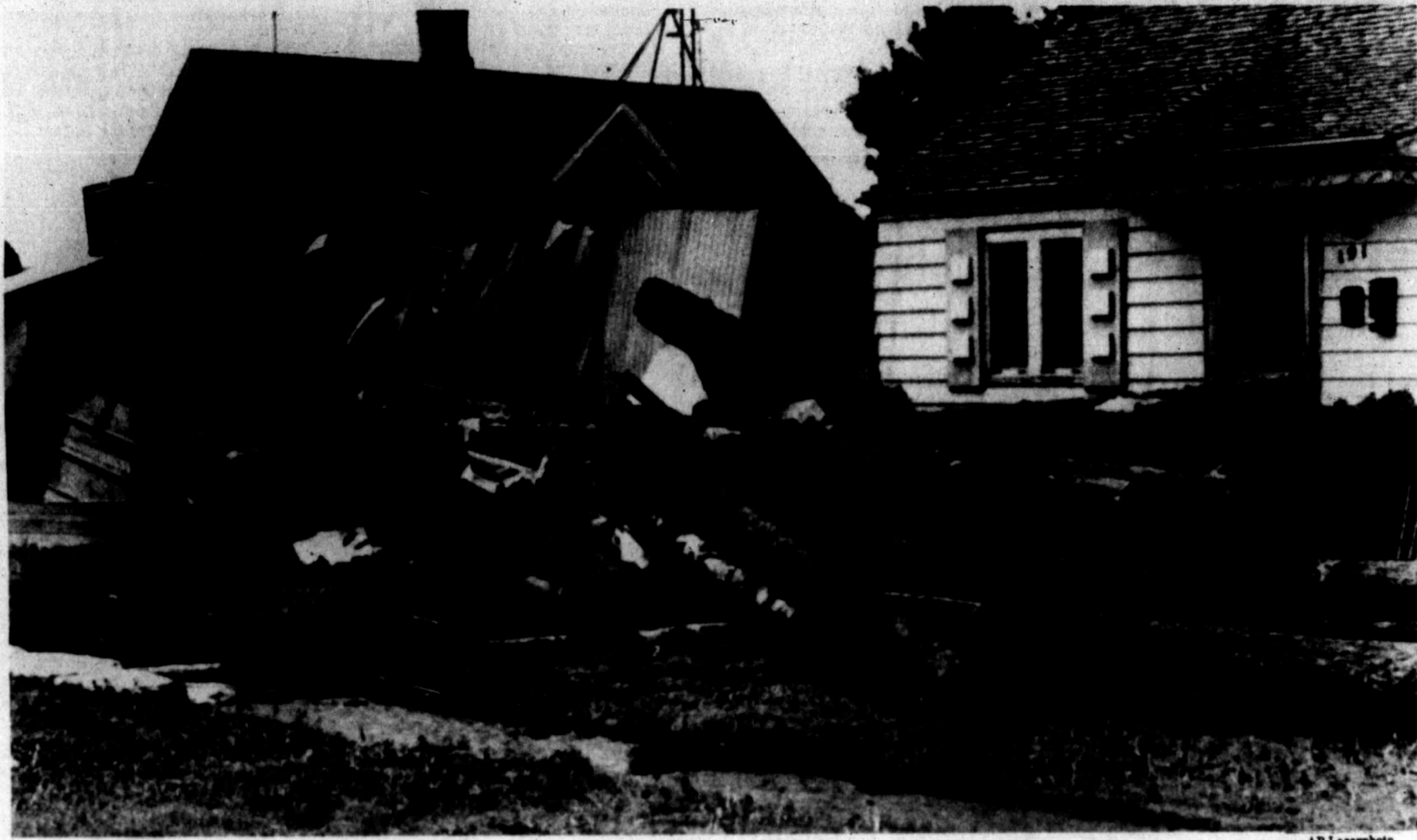
Timber from a nearby lumber yard was carried by the raging floodwaters into this Idaho Falls, Idaho, home and left high and dry collapsed. Evacuations continued today 50 miles downstream from the break.
