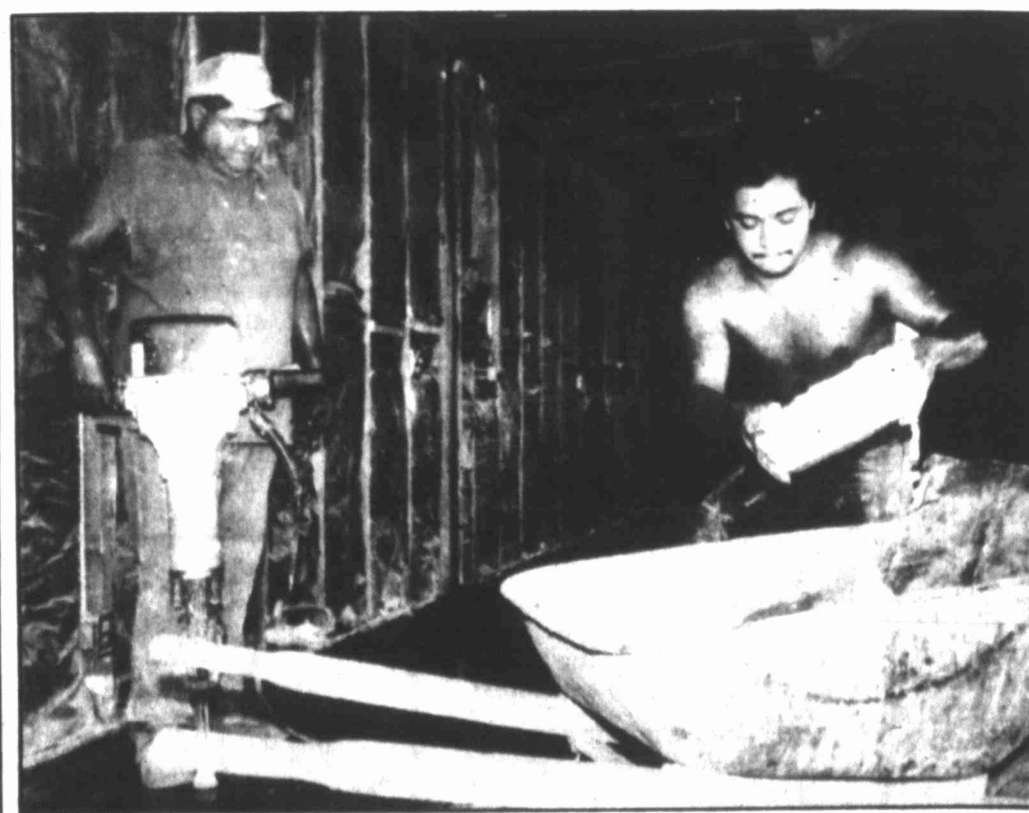
Herald photo by Tim Appel John Cedillos waits as Able Salazar removes chunks of concrete before jackhammering a trench as the two were replumbing the interior of the old Donuts Etc. building in preparation for Little Caesar Pizza.
