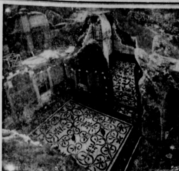
ROME'S NEW SUBWAY UNCOVERS FORGOTTEN MOSAICS —Excavations for Rome's first subway have uncovered ancient Roman apartment houses and public baths deep beneath the central railroad terminal. Workers first came upon old walls which proved to be the fourth floors of residential buildings. The ruins covered several blocks. There were three thermal halls and a heating system belonging to a bathing establishment of the kind popular with the ancient Romans.
