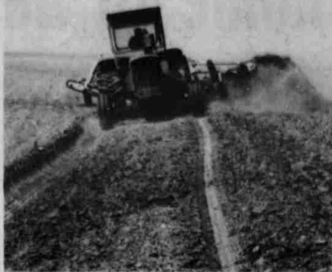
PARALLEL TERRACING — This picture shows parallel terrace construction under way on the U Lazy S Farms, southwest of Post. — (SCS Photo)
