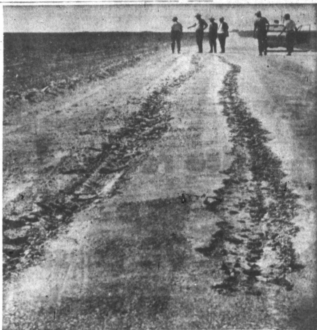
COUNTY PAVED ROADS TAKING BEATING County Commissioners check damage caused by careless plow operators
