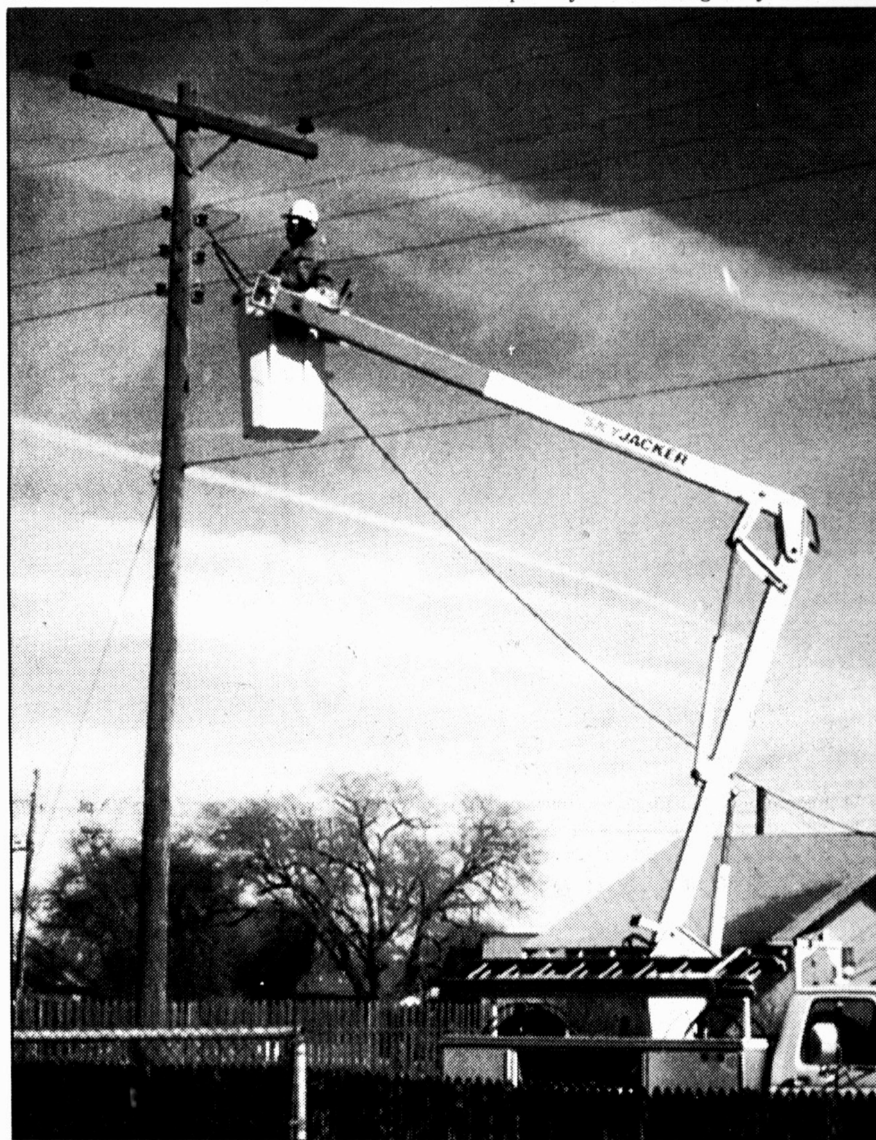
Keeping lines up -- Don Parr, an Southwestern Public Service lineman, checked and replaced some electrical line in the 100 block of Kibbe, Tuesday. Service repairmen have kept busy maintaining lines and doing all they can to guarantee the needed power is available during the cold winter days and even colder nights.
