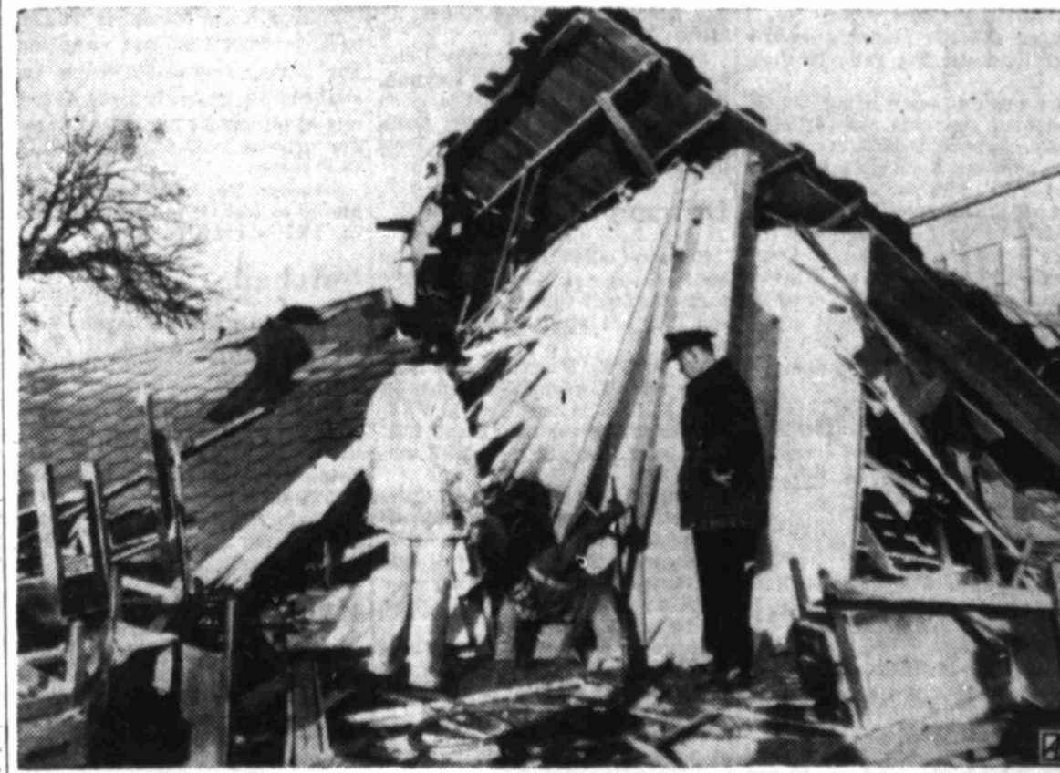
Blast Shatters School Annex
