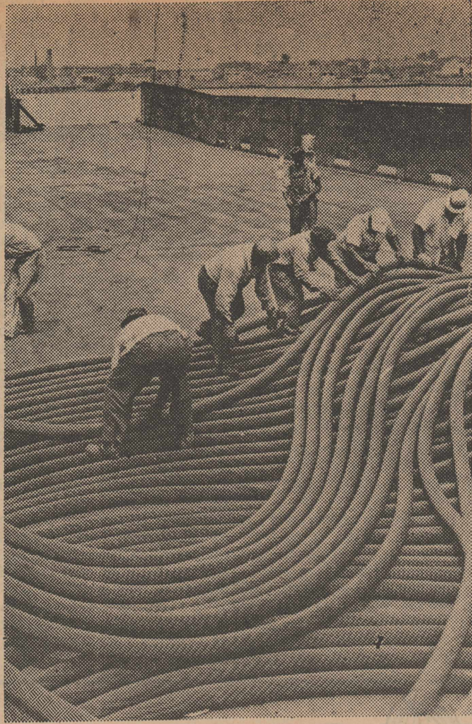
UNDERWATER CABLE —Big loops of steel-armored coaxial cable are unreeling into a barge at Baltimore for the trip that will end under the Hudson River in New York
