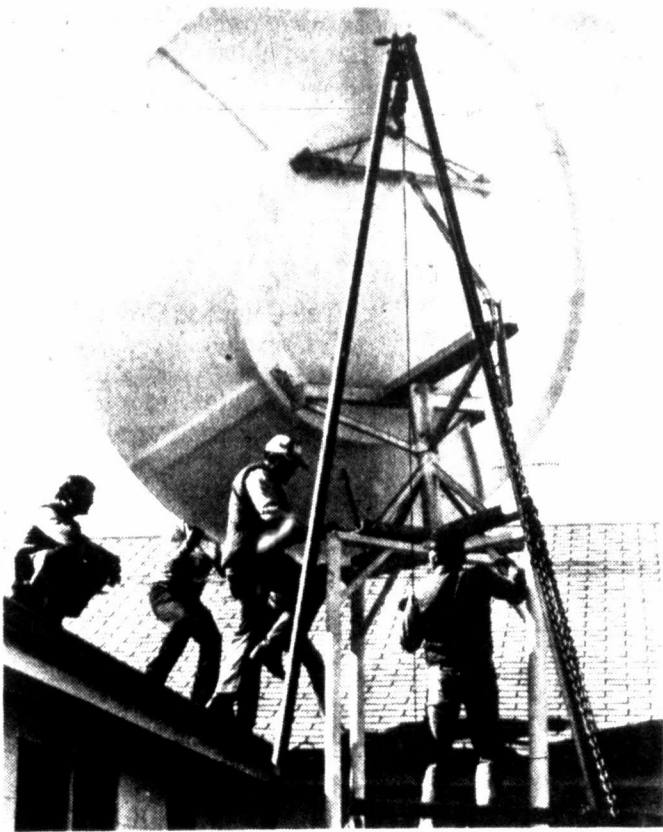
THIS EARTH Receiving Dish, being installed by Mitchell County Broadcasting Company, will afford local Channel Six viewers 24 hour programming. Station owner Joe Kirschbaum (seated left) supervises installation of the dish.
