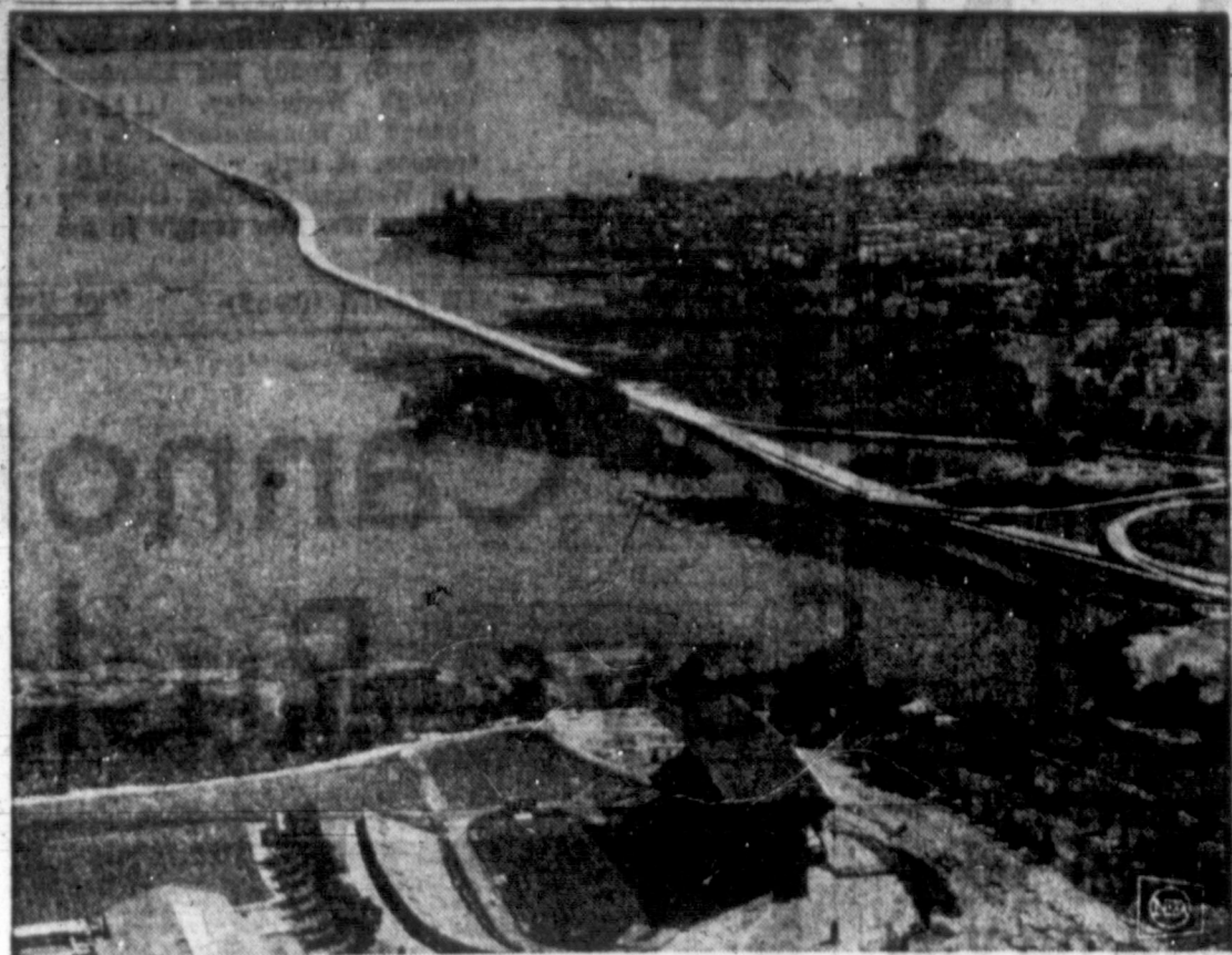
IT FLOATS—Longest floating structure ever built is the newly opened Second Lake Washington Floating Bridge, seen above in a view looking east past the stadium of the University of Washington in northern Seattle. The span, which took three years to build and cost $34 million, crosses more than three miles of water on special pontoons. An earlier floating bridge was built across the southern part of the lake in 1940 and held the world's length record until the new bridge was completed.
